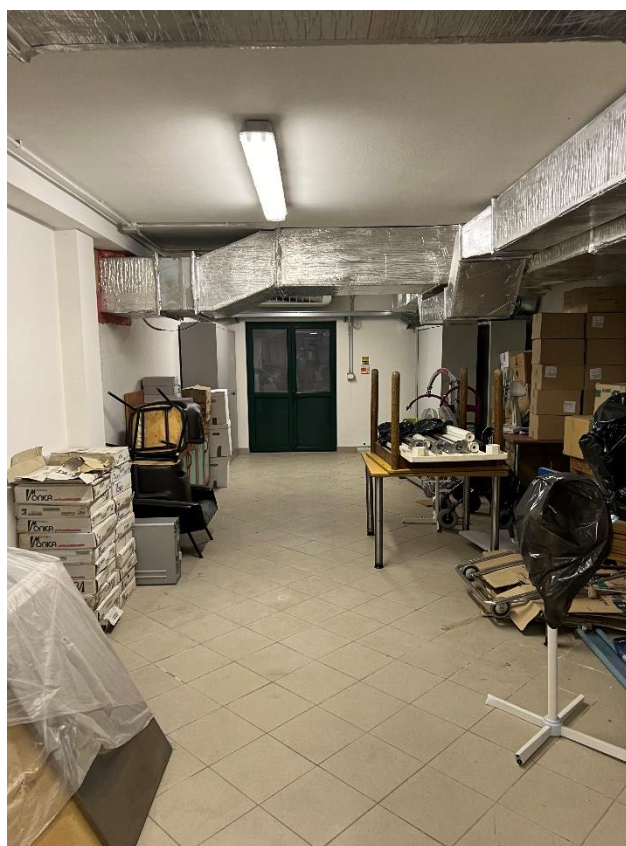
Locale piano interrato
